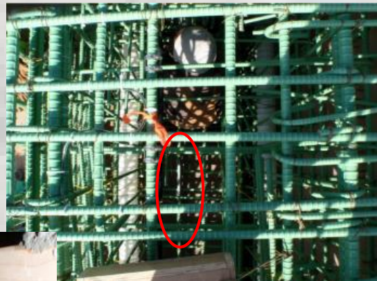
Accelerometer mounting plate and junction box for deck and edge girder arrays.
